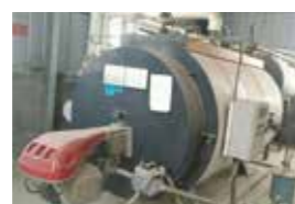
■ Air supply fan for boiler
